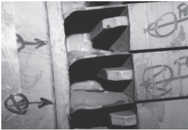
Fig. 6. Defective rotor of a 250kW engine
