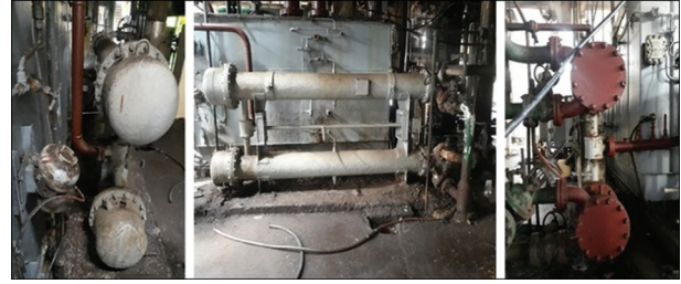
Fig.1. Oil cooler-Type: OKG 33/244
